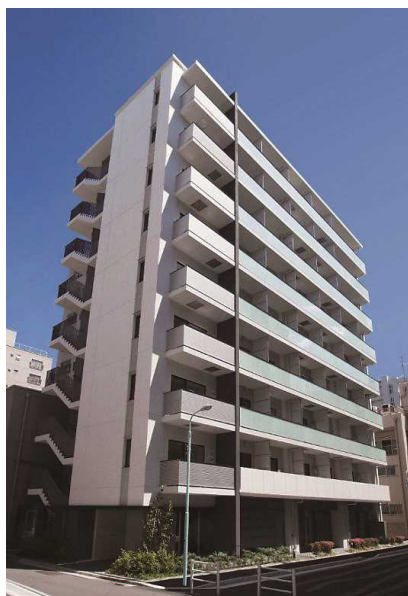
Prime Maison Hatchobori (Location: Hatchobori, Chuo-ku, Tokyo)
